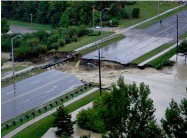
A 2005 storm in Toronto caused $647 million in damages, including destruction of this culvert (left, $4 million) in losses, which was replaced with a larger, more resilient culvert (right). Source: Toronto Environment Office. Photo credit for damaged culvert: Jane-finch.com.
