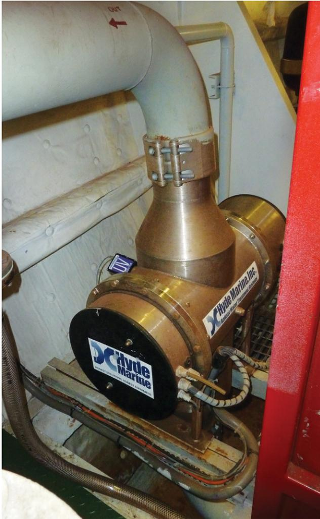
Experimental BWM system enrolled in STEP. In support of USCG, Volpe engineers and marine biologists conduct shipboard visits to observe the BWM system and execution of biological treatment performance experiments.
