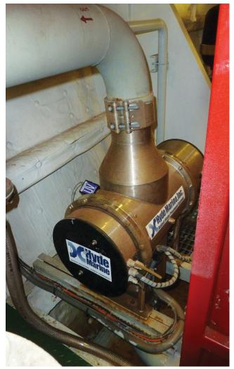
Experimental BWM system enrolled in STEP. In support of USCG, Volpe engineers and marine biologists conduct shipboard visits to observe the BWM system and execution of biological treatment performance experiments.
