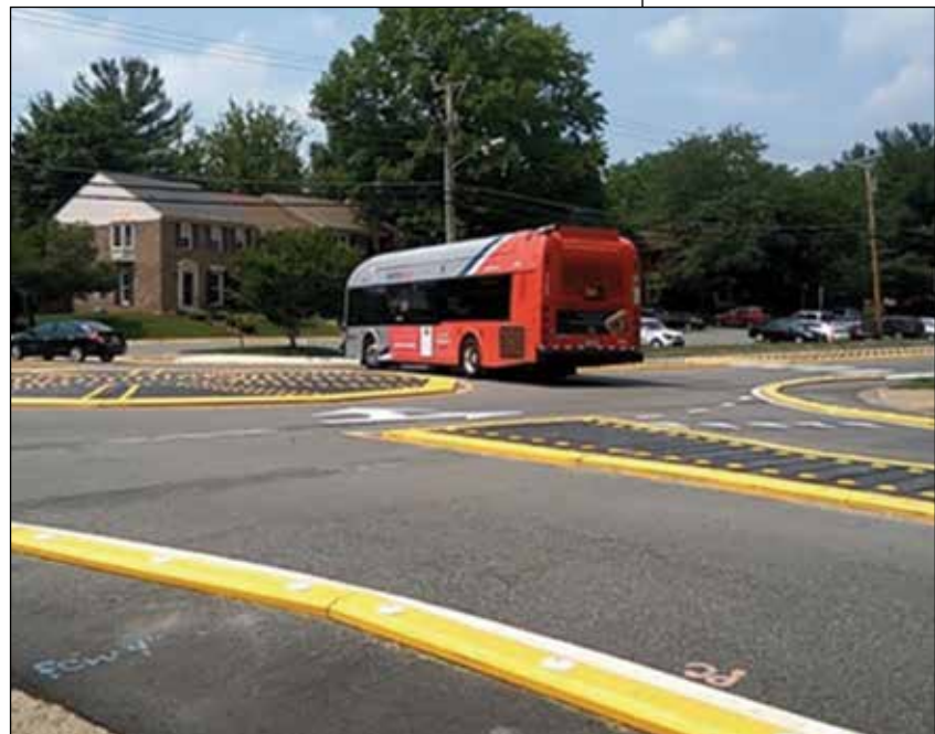
Mini-roundabout, street-level view. (Source: U.S. DOT FHWA)
